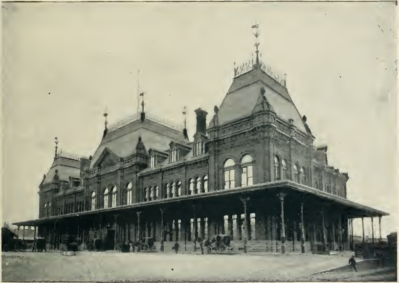
NEW BONAVENTURE STATION, GRAND TRUNK RAILWAY, MONTREAL.
